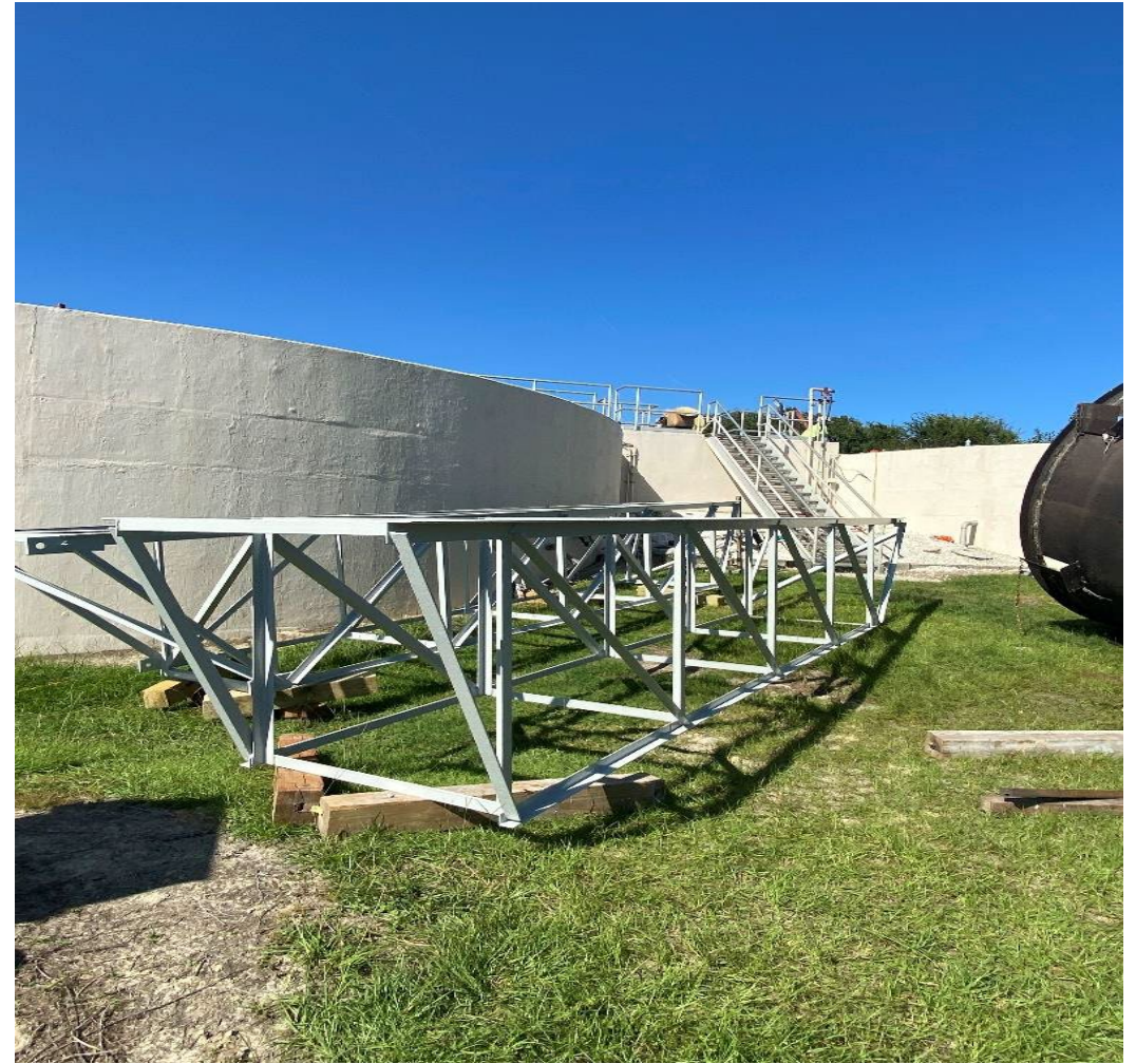
NEW SKIMMERS PARTS PAINTED READY FOR INSTALLATION
