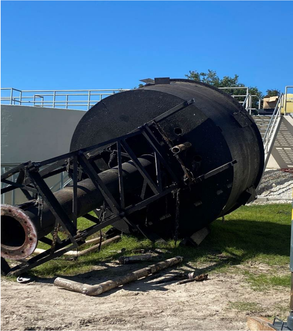
REMOVAL OF OLD FEED WELL
