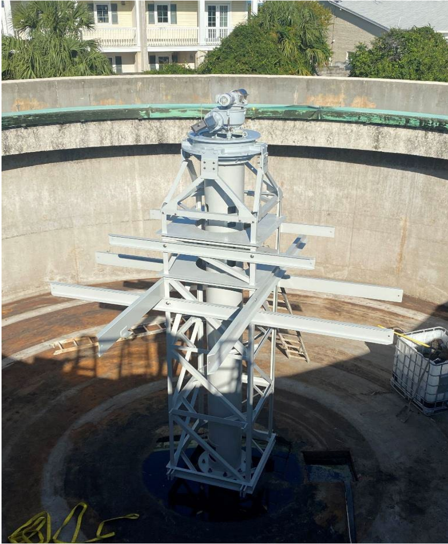
NEW FEED WELL INSTALLED
