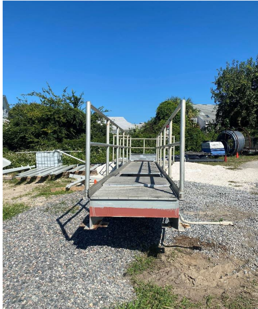
NEW BRIDGE READY FOR INSTALLATION
