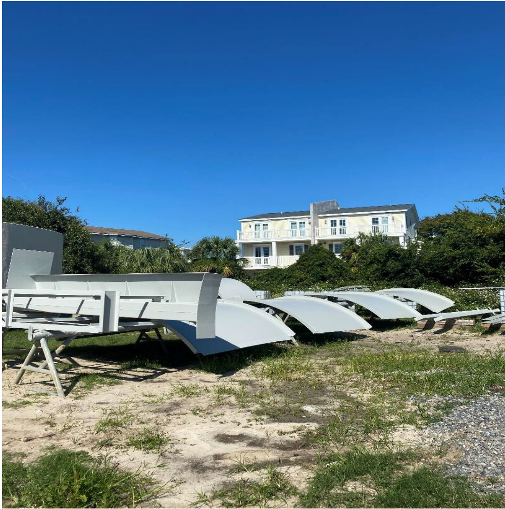
NEW FEED WELL PARTS PAINTED READY FOR INSTALLATION
